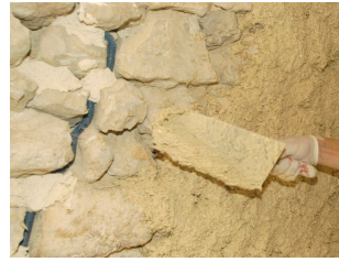
(b) Coating with a trowel ( 800 - 900\ \text{kg.m}^{-3} ).
