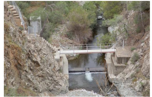
Flow gauging station on Peristerona River near Panayia Bridge. Photo Gerald Dörflinger; date: March 2013
