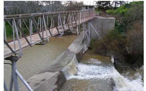
Flow gauging station on Ezousa River near Akhelia. Photo: Gerald Dörflinger; date: February 2009
