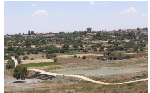
Gabion weir with recharge pond near Orounta village in the lower reach of the river. Photo Gerald Dörflinger; date: May 2013
