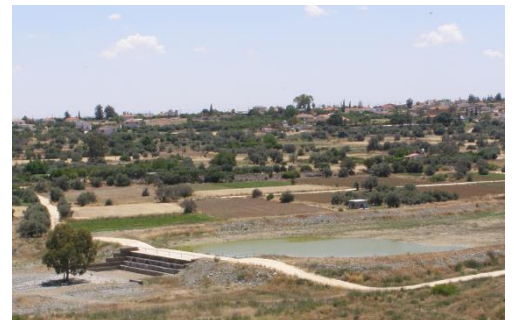
Gabion weir with recharge pond near Orounta village in the lower reach of the river. Photo Gerald Dörflinger; date: May 2013
