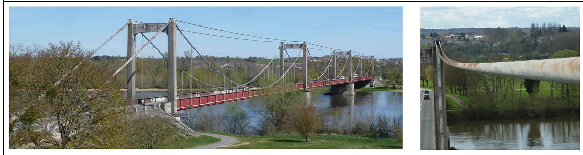
Figure 16. Bonny-sur-Loire (Loiret, France) suspension bridge with top cables.
