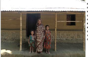
Materials: mud, bamboo, timber Foundations: stone Plinth: stone (main house) & mud (veranda) Columns: reinforced concrete and bamboo posts with or without katla Fences/Walls: mud and Ikar **Roof:** wooden truss, four pitched corrugated galvanised iron sheets Reinforcement: corner bracing **Openings:** 1 main door + 1 inside door to connect rooms Joints: nails, notches, galvanized iron wire Ceiling: protection from heat and cold - rain water harvesting system
