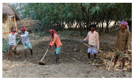
Extraction and preparation of earth for construction
