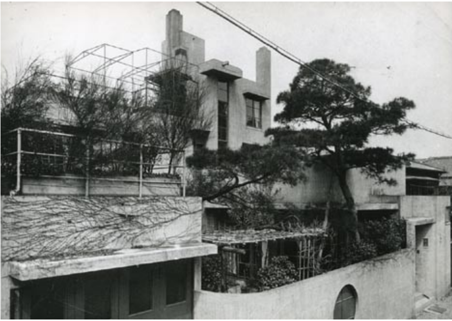
Reinanzaka house, Tokyo, circa 1926. This is the first house Raymond designed for himself and his family. It was made in reinforced concrete in the aftermath of the Great Kantō earthquake that occurred on 1st September 1923. Antonin Raymond archives, Karuizawa. Courtesy of Kitazawa Koichi.
