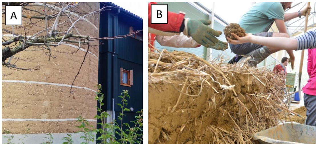
48 Figure 1: A: A rammed earth wall in a building from the 1980's in the Auvergne-Rhone- 49 Alpes region (South-East of France), with clear marks of the layered structure. B: 50 Construction of a cob wall
