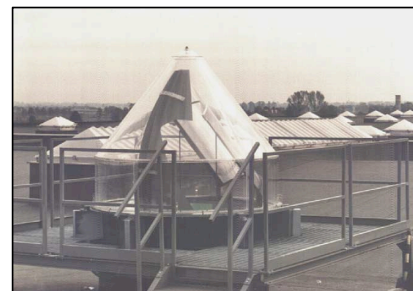
Fig. 13. Active light concentrator Arthelio [37]
