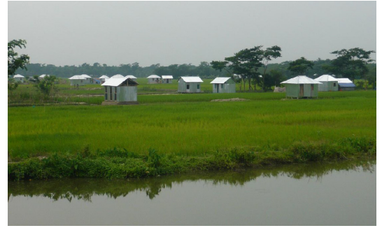
Houses built by NGOs on earthen plinths in paddy field after the cyclone Sidr in Kuakata zone (Barishal). © BUET
