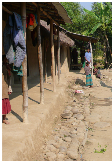
Plinth protection with stones, also used to prevent erosion due to water falling from the roof (Sylhet). ©O. Moles
