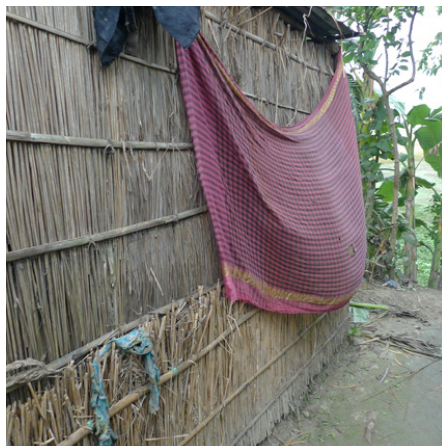
Easy to replace jute stick panels (Rangpur). © A. Caïmi
