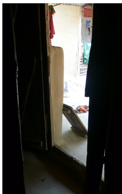
Movable barrier in Sylhet. © O. Moles
