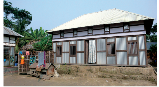
CGI sheet light wall panels in Sirajdikhan (Dhaka). © O. Moles
