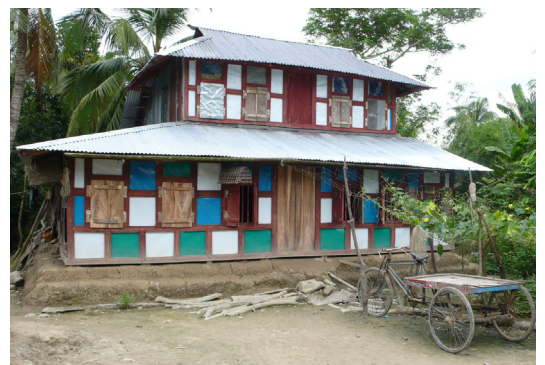
Easily replaceable plywood panels (Barishal). © O. Moles
