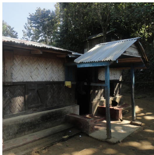
Heavy materials in lower part of the walls (Chittagong). © O. Moles
