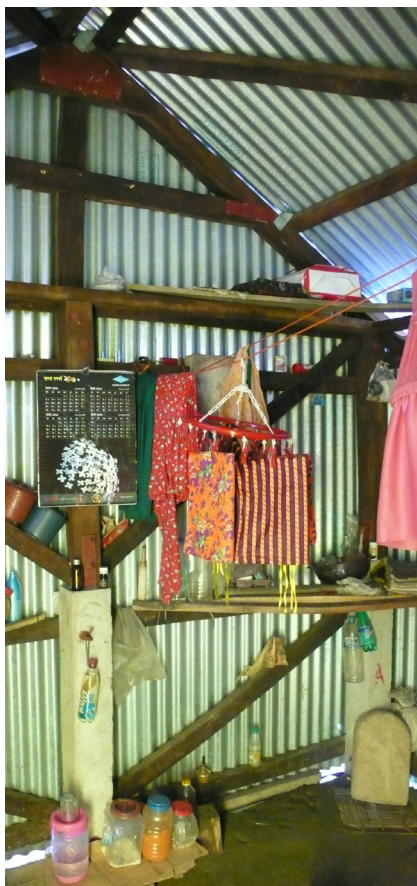
Wooden bracings and katla (concrete plots) in Barishal. Project by DFID and BRAC University. © O. Moles
