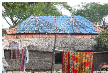
Combined fishing net and bamboo grid in Khulna. © O. Moles
