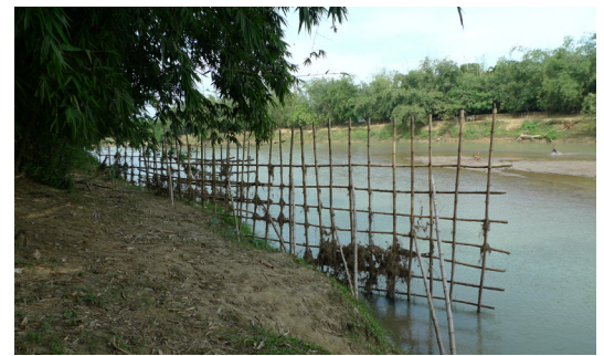
Bamboo grids built on river banks exposed to erosion, working as wave breaker and helping control earth erosion during floods (Mymensingh). © A. Caïmi
