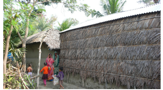
Wall protection according to orientation in Assasuni, Khulna. © O. Moles
