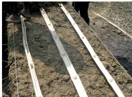
Bamboos are sometimes embedded into cob walls. They improve the behaviour of the wall under horizontal seismic stresses (Rajshahi). © sos-arsenic.net
