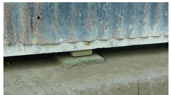
Concrete plots ( katla ) to keep moisture from rising into the wooden structure and gap between walls and soil in Kuakata (Barishal). © O. Moles
