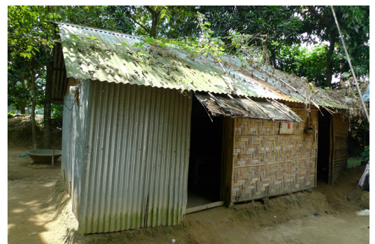
Gap between soil and bamboo wall (Mymensingh). © A. Caïmi
