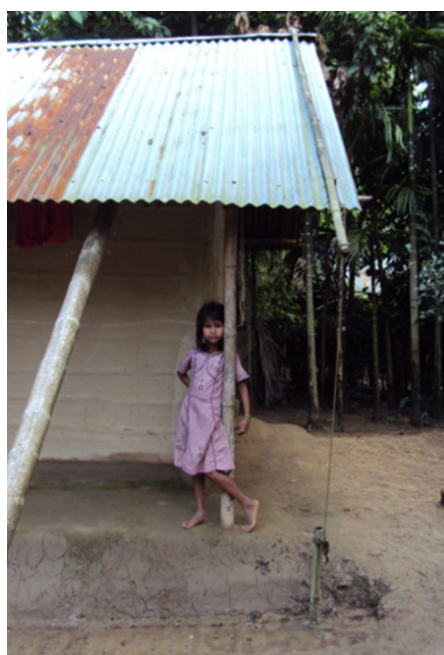
Elevated box platform. © A. Caimi
