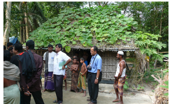
Climbing plants in Kuakata (Barishal) to protect roof from strong winds. © O. Moles
