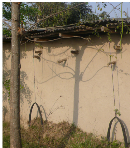
Tyres anchoring in Rajshahi. © O. Moles
