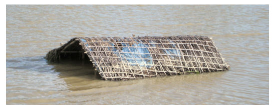
Floating roof. © Unknown
