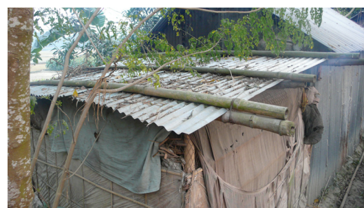
Sheet fastening with bamboo (Rangpur). © O. Moles
