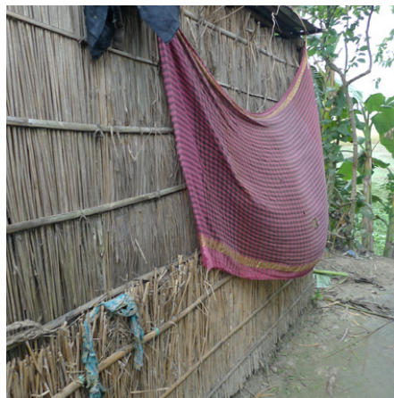
Easy to replace jute stick panels (Rangpur).
