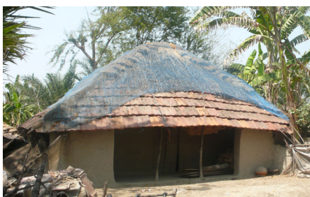
Fishing net for securing the roof in Khulna. © O. Moles
