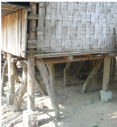
Wooden posts often rely on one or more implanted waterproof elements (Bandarban, Chittagong). © O. Moles
