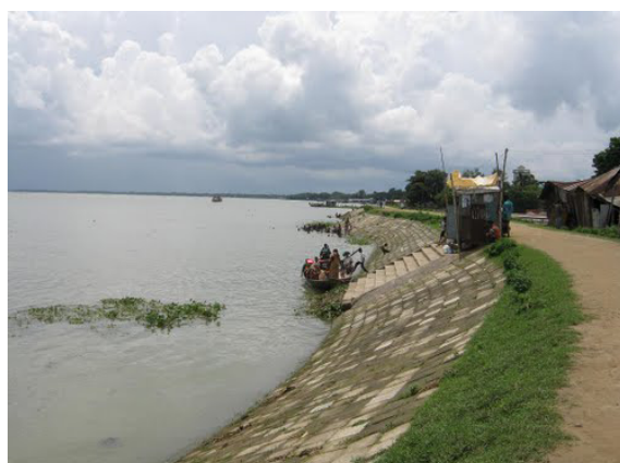
River embankment. © Progress Bangladesh
