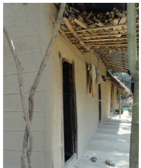
External mezzanine to save goods in flood prone area. © O. Moles
