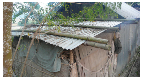
Sheet fastening with bamboo (Rangpur). © O. Moles
