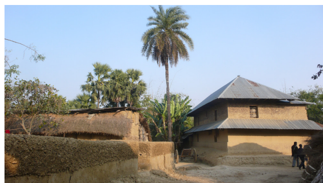
Cob house in progress (left) and finished (right). © O. Moles
