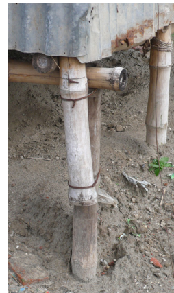
Elevated structure to prevent from soil moisture permeation (Barishal). © O. Moles
