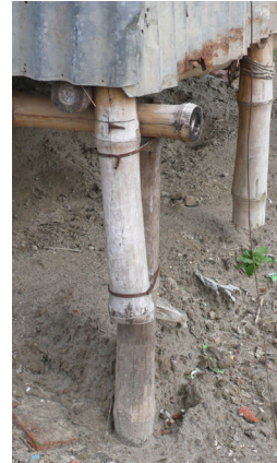
Elevated structure to prevent from soil moisture permeation (Barishal).
