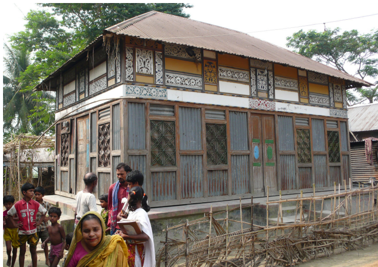
Carved wood and CGI sheet panels in Sirajdikhan. © O. Moles
