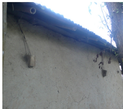
Roof anchoring with fired bricks in Rajshahi. © O. Moles
