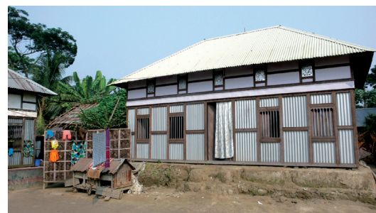
CGI sheet light wall panels in Sirajdikhan (Dhaka). © O. Moles
