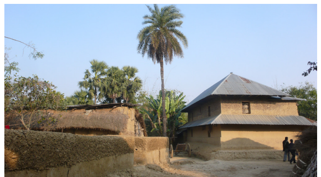
Cob house in progress (left) and finished (right). © O. Moles
