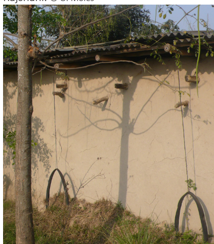
Tyres anchoring in Rajshahi. © O. Moles
