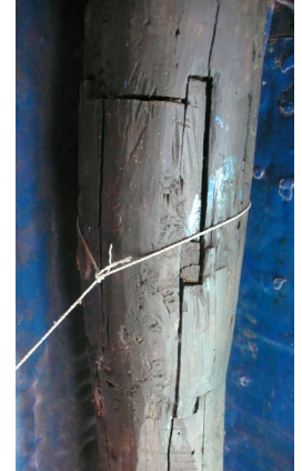
Short separated posts driven into the ground, easily replaceable (Barishal).
