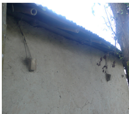
Roof anchoring with fired bricks in Rajshahi. © O. Moles
