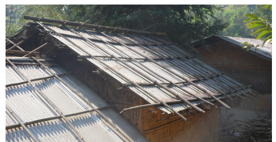
Bamboo grid on CGI roof in Chittagong. © O. Moles
