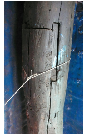
Short separated posts driven into the ground, easily replaceable (Barishal). © O. Moles
