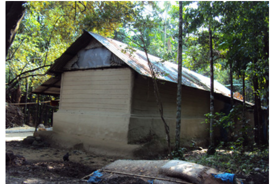
Lower parts of the walls are built with earth (cob), burnt bricks or cement blocks, and upper parts with reed mats, bamboo mats or iron panels (Sylhet). © O. Moles
