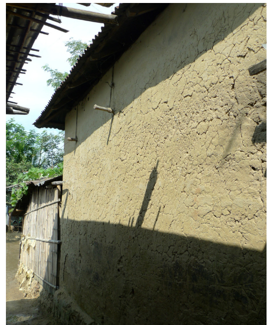
The roof is tied to bamboo pieces embedded through the walls (Mymensingh). © A. Caïmi
