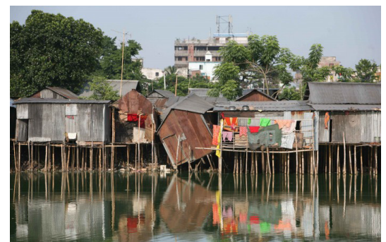
Stability problems in slum houses in Dhaka, Bangladesh, raised above ground level to protect against flooding. © Manoocher Deghati/IRIN
