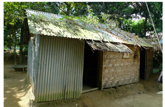
Gap between soil and bamboo wall (Mymensingh).
