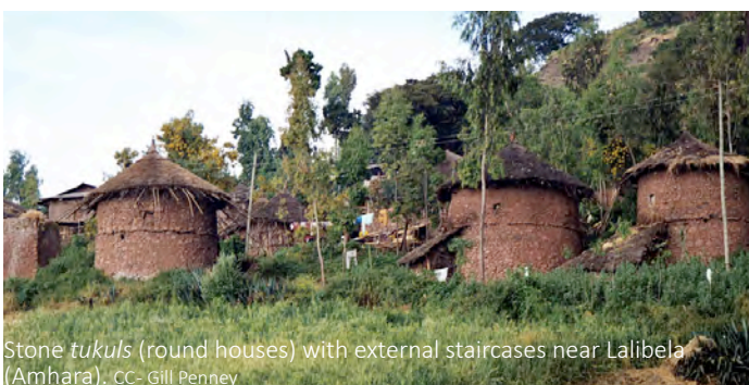
Load bearing stone masonry walls in Tigray CC - Rod Waddington
