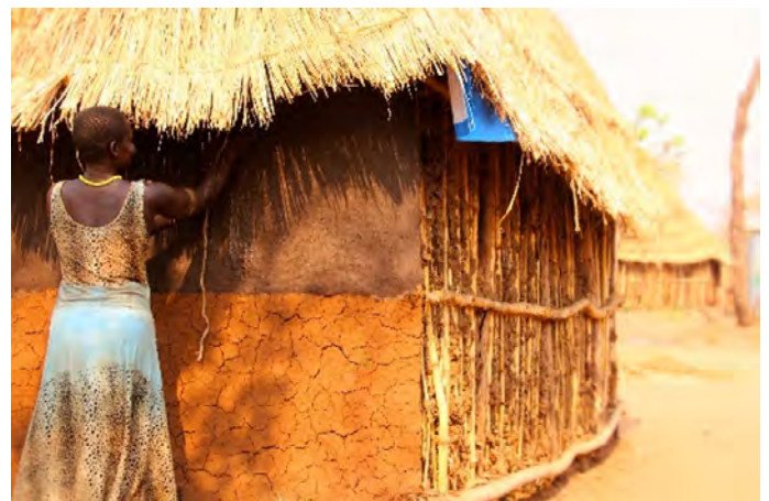
Active participation of beneficiaries through mud plastering and thatching. © Muse Mohammed - IOM
