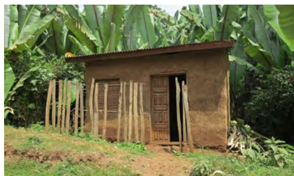
Chikka house in Gedeo Zone (SNNPR). © ShelterBox
