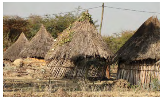
Stability problems due to black cotton soil expansion and contraction near lake Tana (Amhara). © L. Davis
