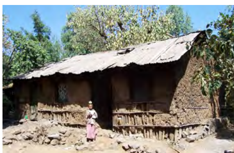
Chikka rectangular house with CGI sheet roofing in Felasha village, near Gondar. CC- Beth
