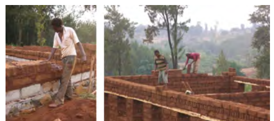
Adobe construction in Aira (Oromia). © Petersson & Ström
