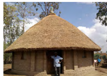
Earth from termites nests is used by the Alaba people for good quality durable plasters. The house in the right has been built with earth from termites nests. (Oromia-SNNPR). © Lorenzo Fontana
