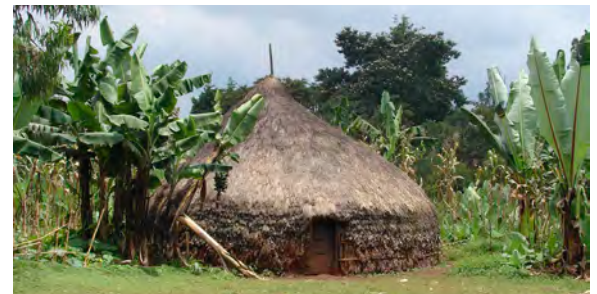
Sidama people house built with a bamboo structure and a vegetal covering for walls and roof. cc- Maurits Vs.
