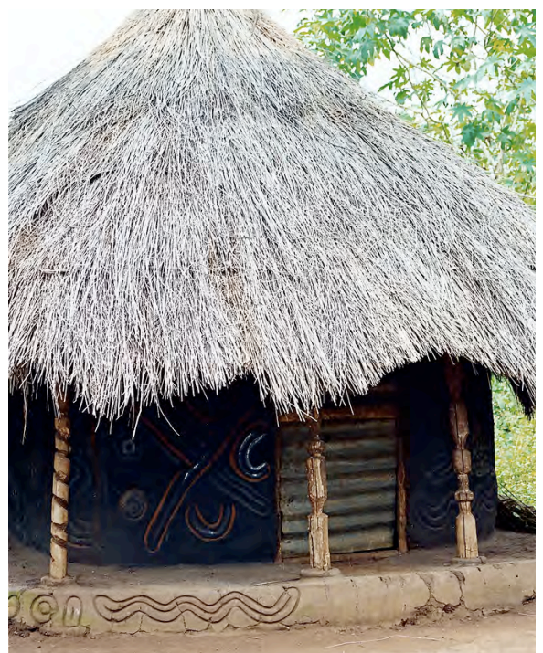
Anuak house on an earthen mound, with verandah and mural paintings in Gambela. CC- Gill Penney
