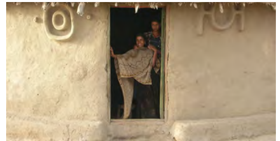
Earthen plinth in an Alaba house (SNNPR). © Lorenzo Fontana
