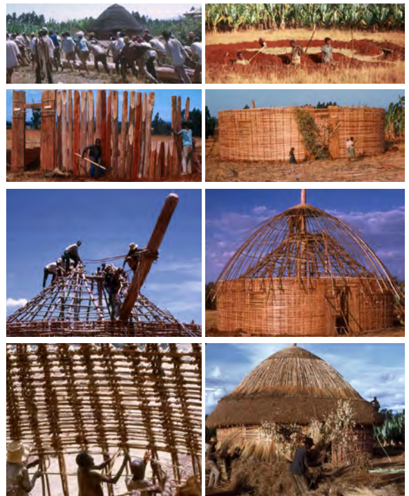
Collective construction of a Gurage house. © Michael Santarelli
