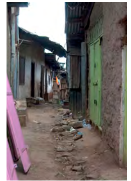
Stones forming a gutter to avoid soil erosion when water falls from roofs. Addis Ababa. CC- PicturesFromWords
