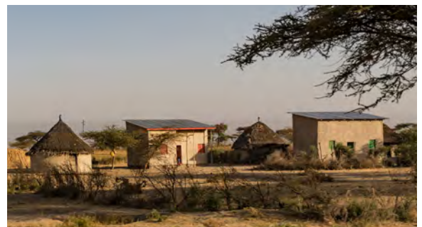
Rectangular houses with CGI sheet roofs and round houses with thatched roofs, both with chikka walls near Langano lake, Oromia. CC- Ninara
