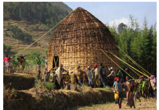
Dorze house being moved by the whole community in SNNPR. Bamboo structure is visible. © H. Mengitsu
