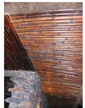
Bamboo ceiling near Bura (Amhara). Ceilings improve the house's comfort. © O. Moles- CRAterre
