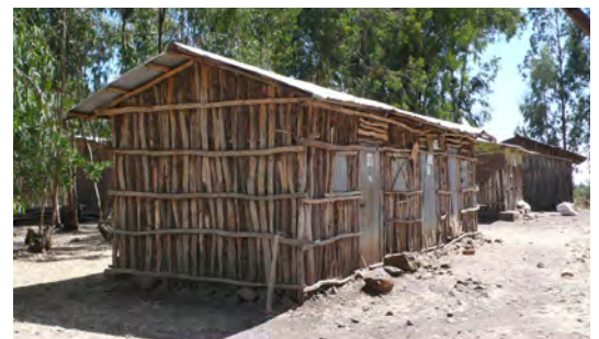
Flexible wooden construction in a black cotton soils area in Bahir Dar (Amhara). © O. Moles- CRAterre
