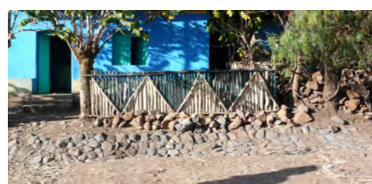
Surface drainage system to prevent from erosion and flooding near Bahir Dar, Amhara. © O. Moles
