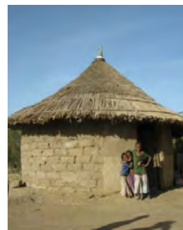
Adobe round house in the Ethiopian Rift Valley (20 years since construction). © Petersson & Strom
