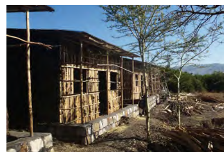
New chikka houses under construction in Amhara region. CC- Canned Muffins
