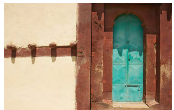
Church of Abba Afse with «monkey heads» technique in the walls. Yeha, Tigray. CC- A. Davey
