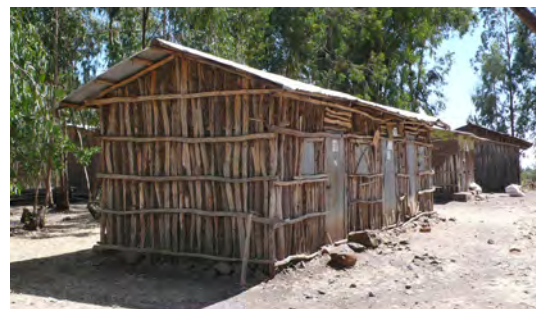
Flexible wooden construction in a black cotton soils area in Bahir Dar (Amhara). © O. Moles- CRAterre
