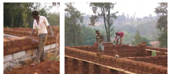
Adobe construction in Aira (Oromia). © Petersson & Ström
