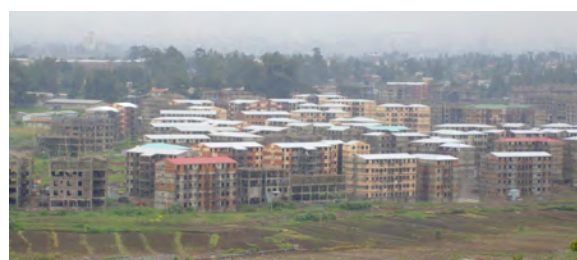
Condominiums under construction Addis Ababa. CC- Maguns Franklin
