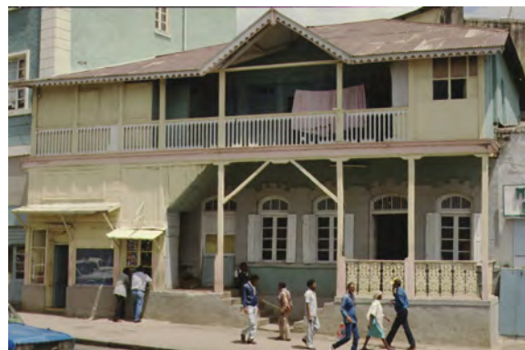
Addis Ababa style building with verandah. ©T. Joffroy-CRATERE
