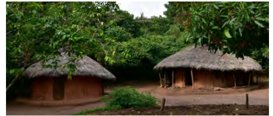
Aari houses built on a mound with a round verandah protecting the walls from the rain. (Debub Omo Zone in SNNPR). CC- Richard Mortel
