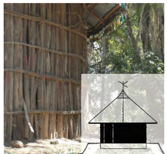
This church (Bura, Amhara) lies on an earthen mound to protect against floods. There is a corridor between the interior earth wall and the wooden exterior wall. These two elements prevent from the effects of black cotton soils expansion if the platform is built with inert earth, and so cracking of walls is avoided. © L. Davis
