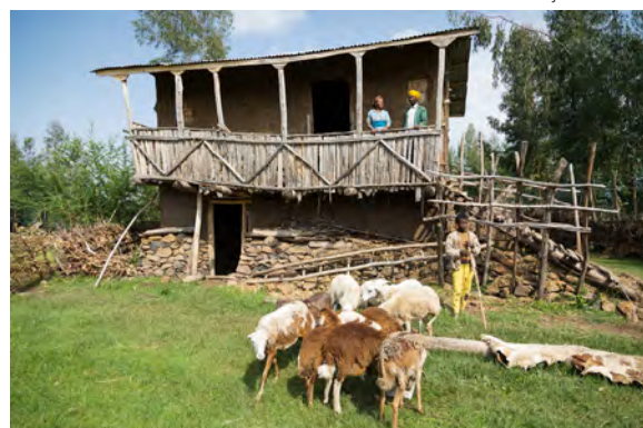
Two story house with stone plinth, chikka walls and balcony in Gogbob village, Amhara region. CC- Kelley Lynch USAID
