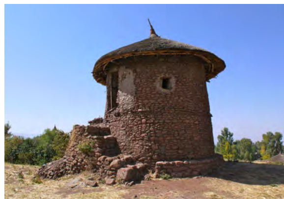
Stone tukul in Lalibela with two levels and exterior staircase. CC- Martijn Munneke
