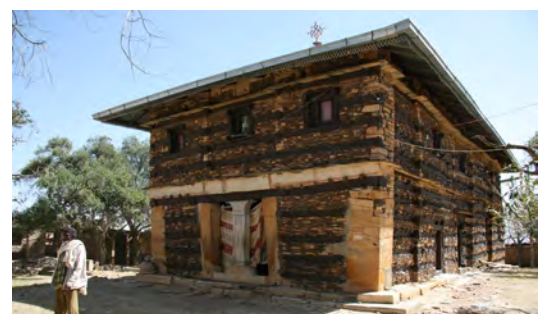
Church with horizontal «seismic» timber bands or «monkey heads» in Debre Damo monastery in Tigray. CC- Travel Aficionado
