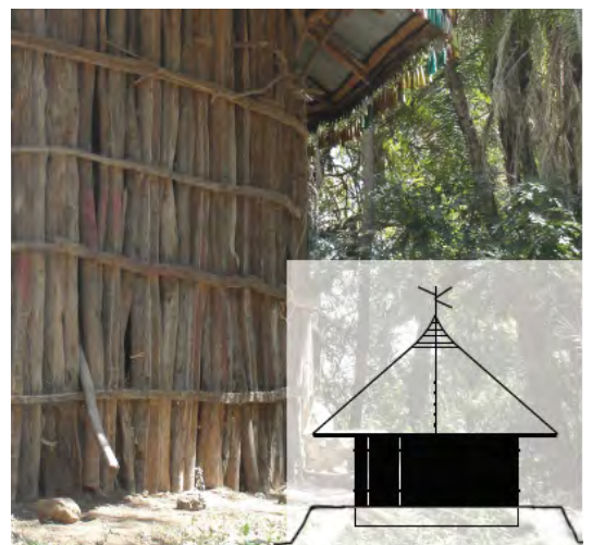
This church (Bura, Amhara) lies on an earthen mound to protect against floods. There is a corridor between the interior earth wall and the wooden exterior wall. These two elements prevent from the effects of black cotton soils expansion if the platform is built with inert earth, and so cracking of walls is avoided. © L. Davis
