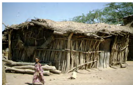
Permanent constructions with wooden structure and earthen roof in Afar region. ©T. Joffroy- CRAterre
