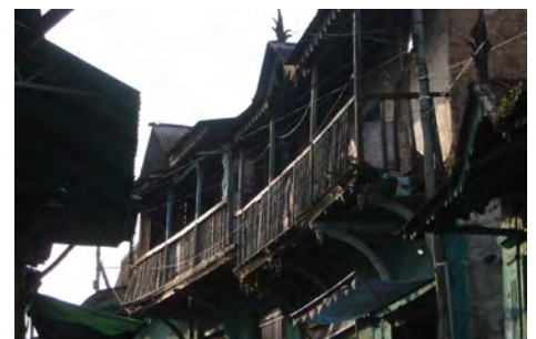
Balconies in the city centre. CC- Ahron de Leeuw
