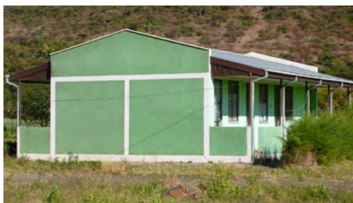
Contemporary construction made of elements disconnected from each other is a good practice for the building not to crack due to black cotton soil expansion and retraction. Near Bahir Dar, Amhara. © O. Moles- CRAterre
