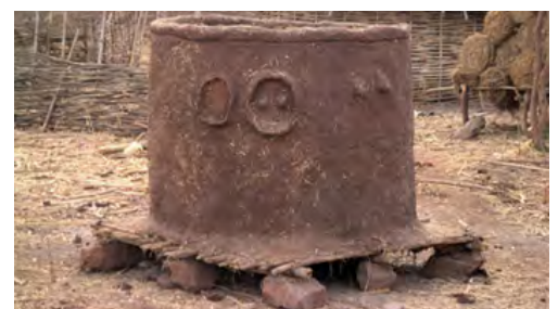
Raised Gumuz clay granary on a platform of branches placed on top of stones or directly on stilts. Manjari, Metekel Zone. CC- González Ruibal
