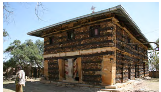
Church with horizontal «seismic» timber bands or «monkey heads» in Debre Damo monastery in Tigray. CC- Travel Aficionado
