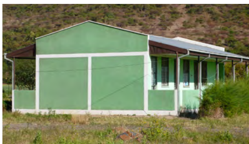
Contemporary construction made of elements disconnected from each other is a good practice for the building not to crack due to black cotton soil expansion and retraction. Near Bahir Dar, Amhara. © O. Moles- CRAterre
