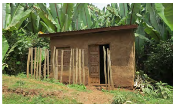
Chikka house in Gedeo Zone (SNNPR). © ShelterBox
