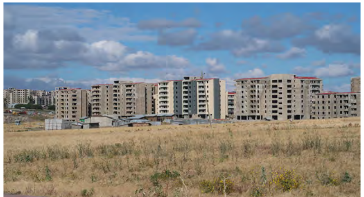
Condominiums under construction in Addis Ababa. © V. Murtagh
