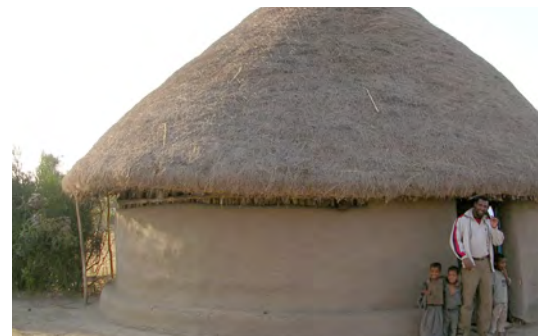
Ventilation is made possible thanks to the absence of plaster in the upper part of the walls in the Alaba houses (SNNPR). © Lorenzo Fontana
