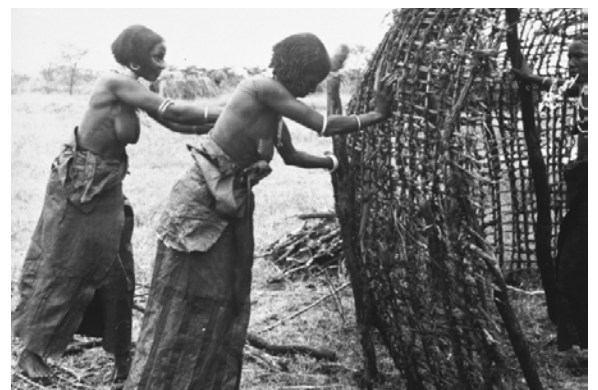
Construction of a Borana «bird's nest» house. CC- National Museum of World Cultures
