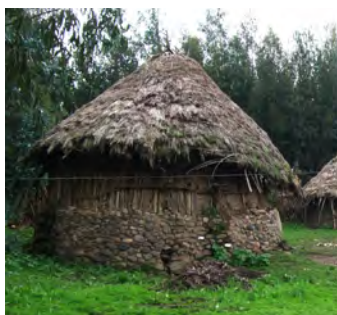
Constructions with stone plinths for protection of the wood and chikka walls from moisture and water splashing on the walls. (Amhara).
