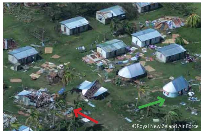
CI sheet bure after cyclone Winston: even if some have been damaged, they have resisted better than other constructions.
