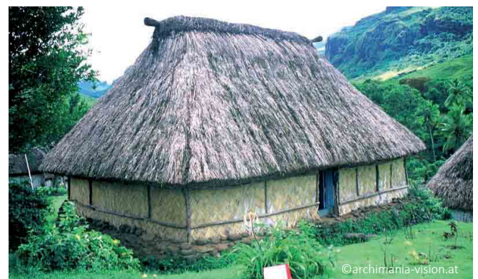
Traditional house: woven mat walls are fixed on the outside with additional wood elements to improve resistance to wind pressure; the top of the roof is reinforced with an additional layer of special grass tied to a timber beam protruding from two sides of the roof.
