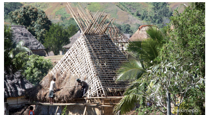
A net of woven reeds is applied on the rafters to better fix the thatching.
