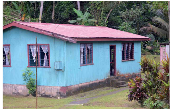
Formal timber-framed house on cement block plinth.
