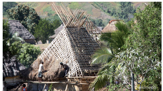
A net of woven reeds is applied on the rafters to better fix the thatching.
