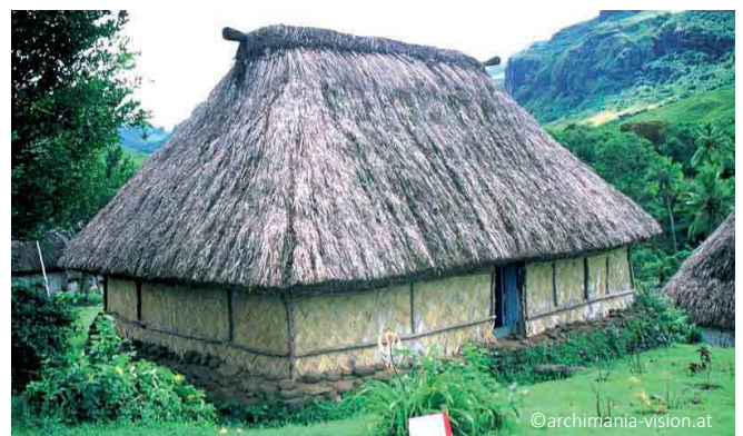
Traditional house: woven mat walls are fixed on the outside with additional wood elements to improve resistance to wind pressure; the top of the roof is reinforced with an additional layer of special grass tied to a timber beam protruding from two sides of the roof.
