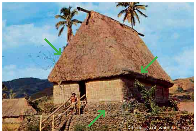
Elevated stone platform for protection from floods and soil erosion. Small eaves and steep roof for reduced vulnerability and improved durability.
