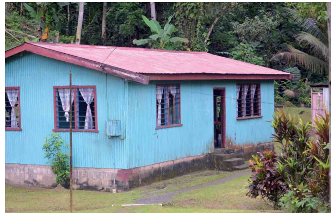
Formal timber-framed house on cement block plinth.
