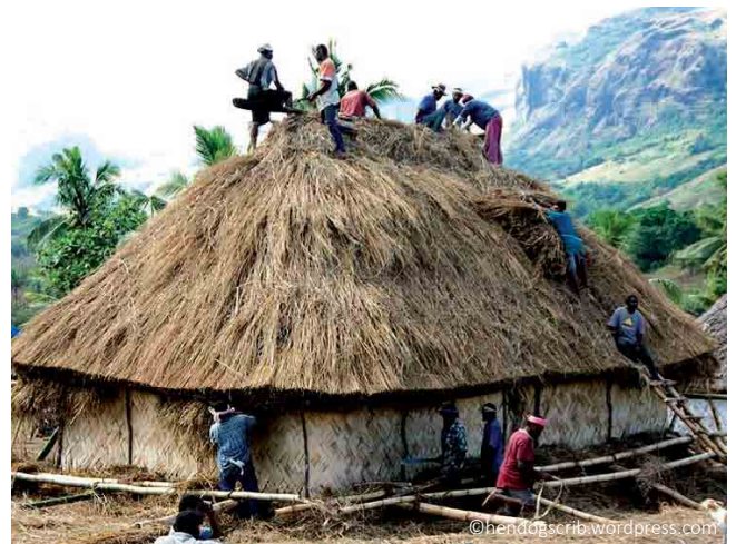
Housing construction with the involvement of the community.
