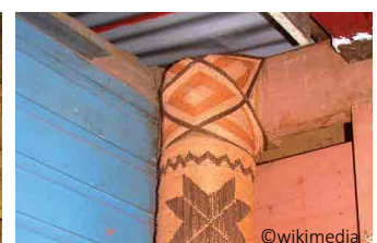
Coconut fibre tying for roof trusses (left) and corner post-ring beam (right).
