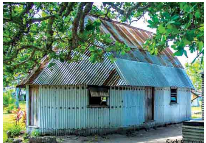
Bure built using CI sheets as evolution of the traditional building practices: round shape for improved aerodynamicism.
