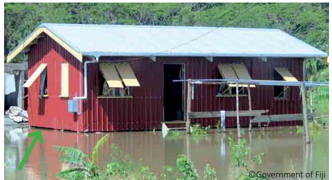
Elevation of the house above ordinary flood level.
