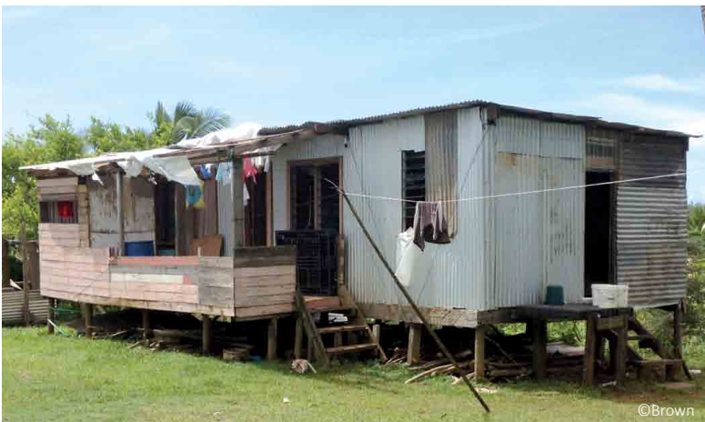
Precarious sheet housing: elevation on stilts for better protection from floods.
