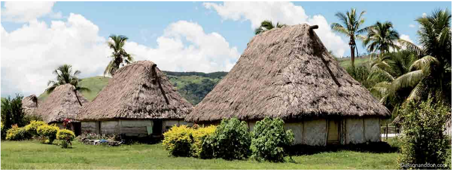
Vernacular housing: lightweight flexible construction and 4-slope hipped roof for better wind resistance.
