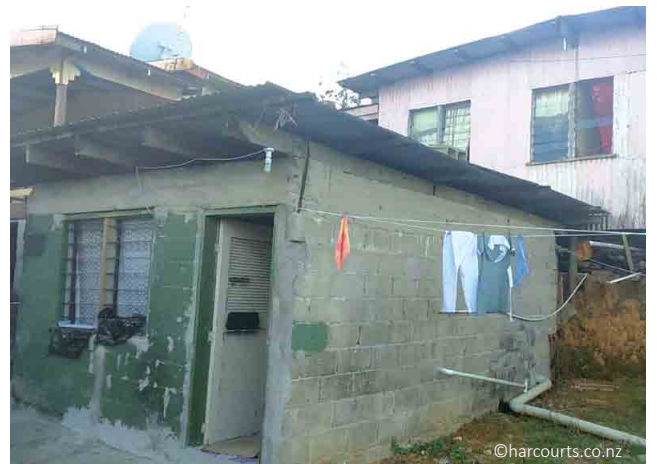
Formal low-cost housing result of global influences: cement block masonry with anchoring for roof structure.
