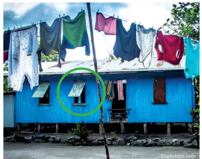
CI sheet house: tilting shutters can be easily fixed during cyclones. ©selcitron.com
