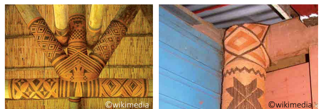
Coconut fibre tying for roof trusses (left) and corner post-ring beam (right).
