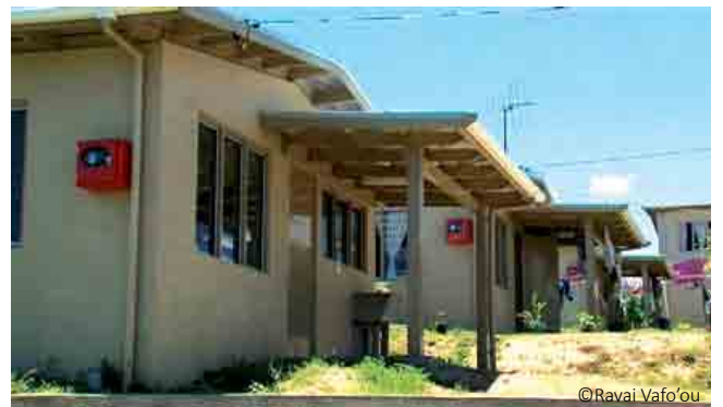
Government-subsided low-cost housing. ©Ravai Vafo'ou
