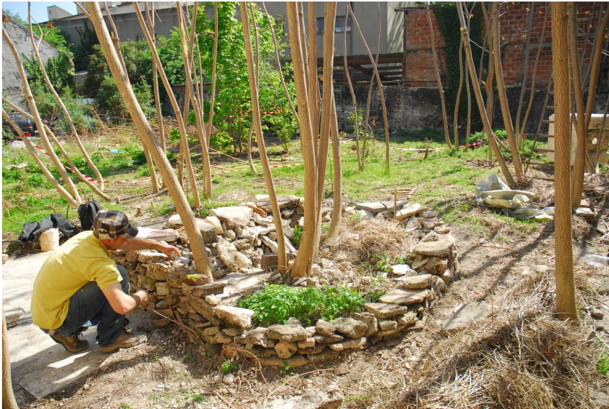
Figure 10.3: Léonard Nguyen Van Thé builds a dry-stone wall around a tree of heaven ( Ailanthus altissima ) on a brownfield site in Aubervilliers. The pit will later be filled with vegetable waste and dry leaves to make a bateau—a walled lasagna. Photo by Jens Denissen.
