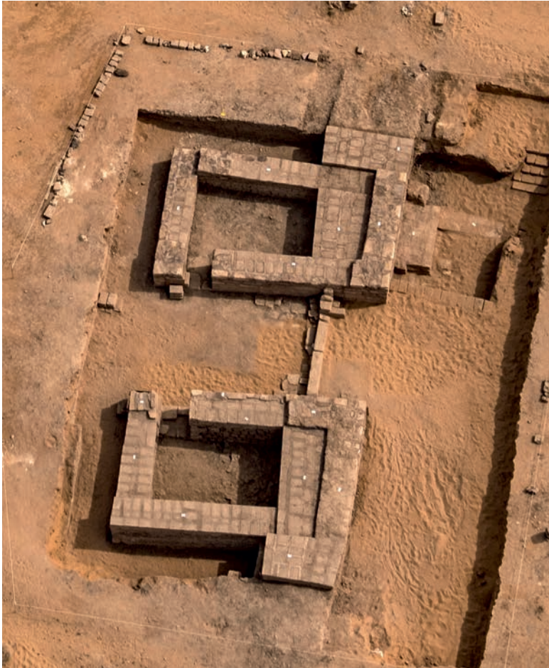
Fig. 2. Aerial view of the South-east gate after restoration.
