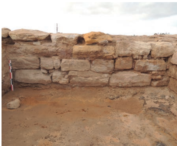
C. Northern facing of wall 60880.
