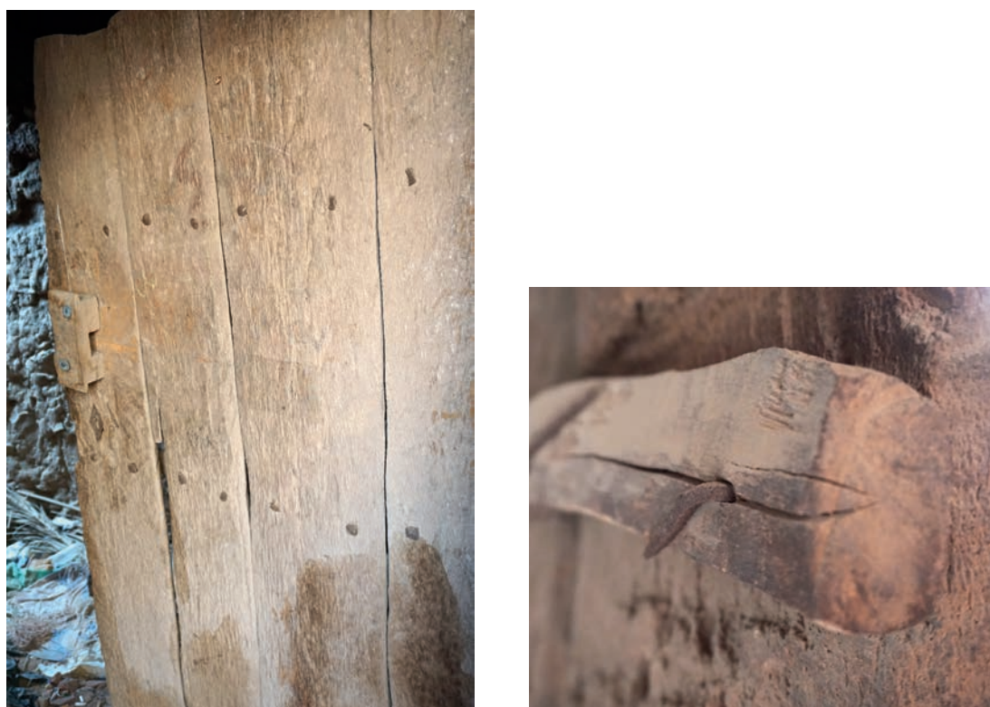
Fig. 2. Modern door in the old city of al-'Ulā, made of several sections of date palm trunk (a) joined together with a transversal beam (Tamarix) and nails (b).
