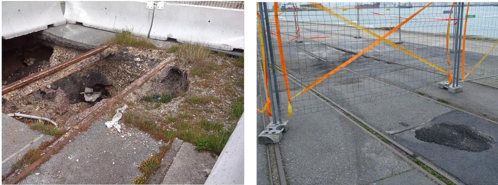
Figure 2: Photo of typical collapse and deformation observed these last years on the Joannes Couvert quay.
