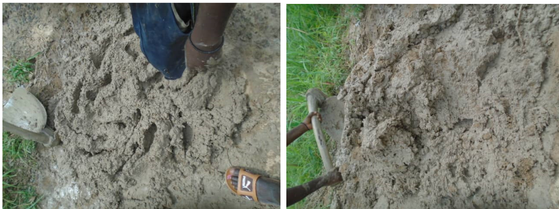
Figure 3: Wet Heap Mixed to become Viscous
