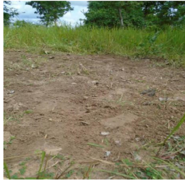
Figure 2: Cleared Ground for laying Bricks
