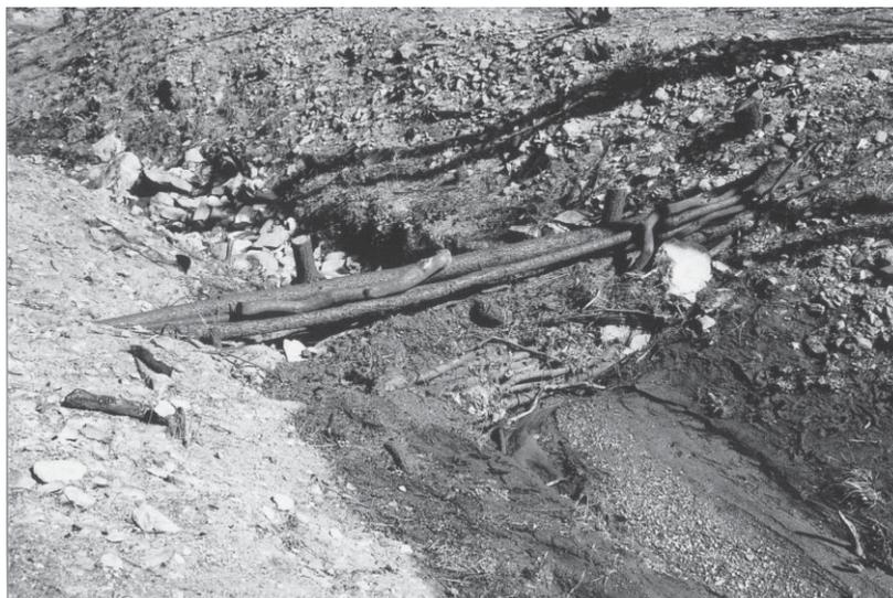
**Figure 2.** Log debris dam (LDD) showing trapped sediment and debris upstream of dam.
