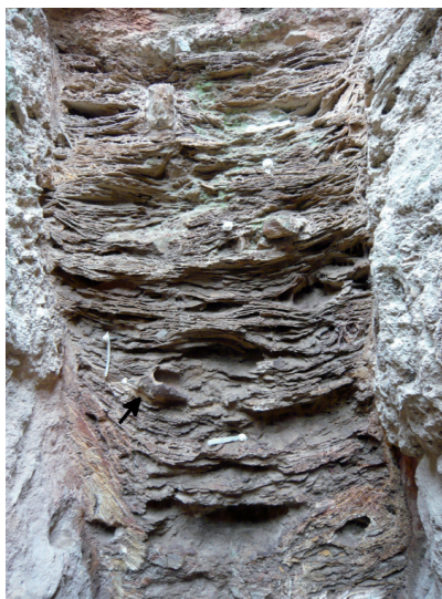
Figure 4: Puff-pastry travertine filling the aqueduct at Jebel Oust, Tunisia. The black arrow indicates an archaeological element encrusted in the precipitated sediment; the channel is about 1 m wide.
