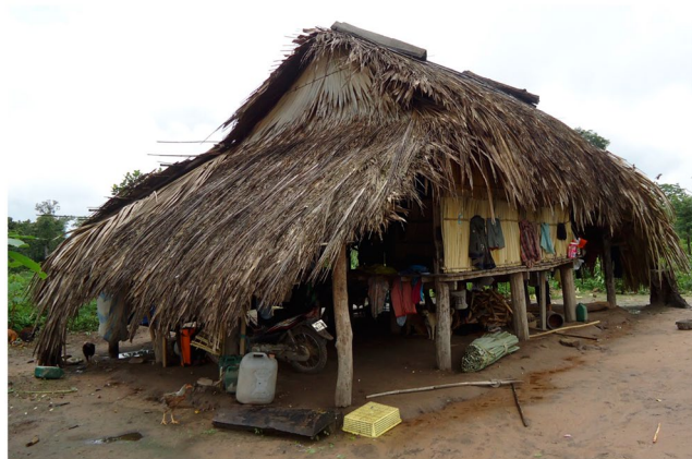
Figure 2. Example of different housing styles in the study villages. Panel A: Ground-level house constructed of wood walls and floor, and tin roof. Panel B: Elevated house constructed of bamboo walls and floor, and plant-based (palm frond) roof. Photographs taken by author Set Srun.
