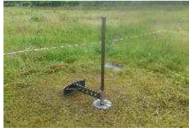
Preparation of a trench for the ground anchoring of the box
