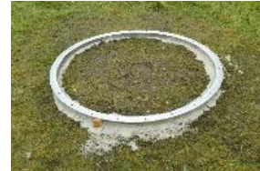
Installation of a skirt for anchoring the chamber
