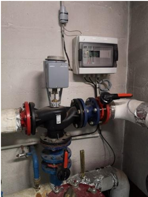
Figure 1: Installation example of a thermal energy meter for heating energy demand monitoring
