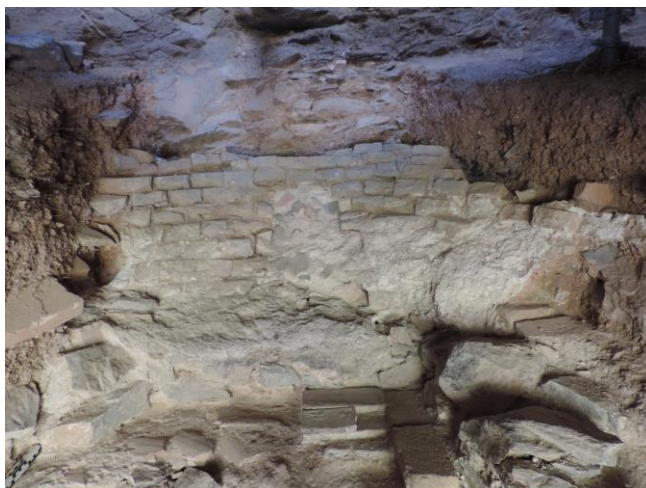
Fig. 6 Gypsum plaster restorations in the bottom of the furnace (cl. D'Ovidio A-M)
