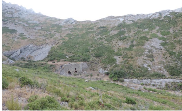
Fig. 1 Valley of the Panouse: quarry, lime kiln and grappier (cl. D'Ovidio A-M)
