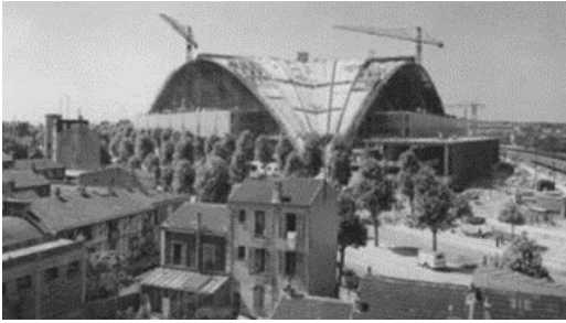
Fig. 1 The CNIT under construction
