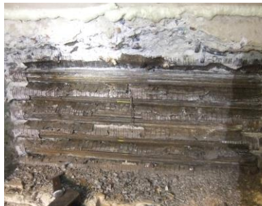
Fig. 12. Good conservation of the wires after removal of the ducts
