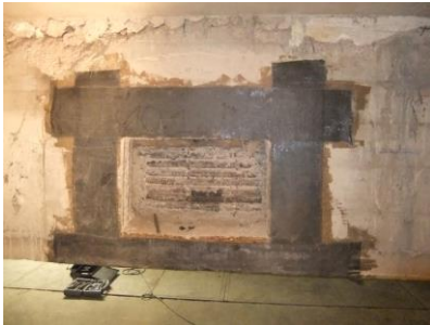
Fig. 11. Opening of a window in the tie after a local strengthening by CFRP.
