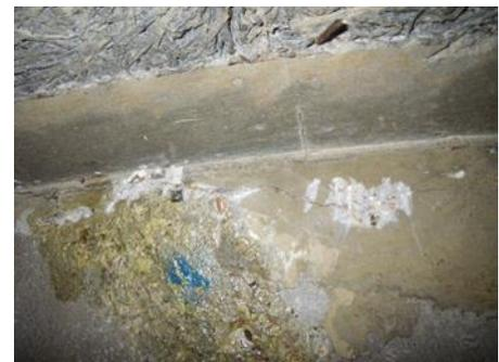
**Fig. 10.** Example of cracks located in the patch repair at diaphragm/shell junction.
