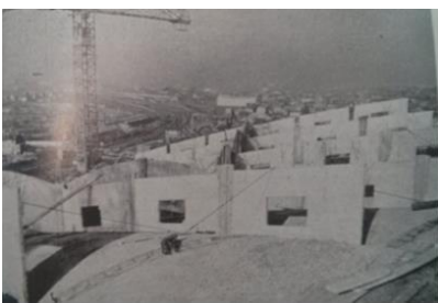
Fig. 5. View of the lower shell, webs and diaphragms.
