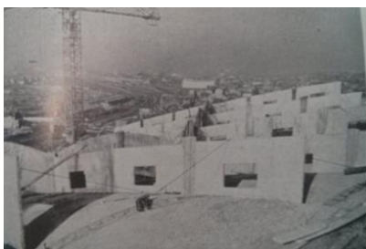
Fig. 5. View of the lower shell, webs and diaphragms.
