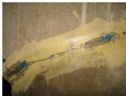
Fig. 9. Example of an injected crack detected in the diaphragms of the vault.
