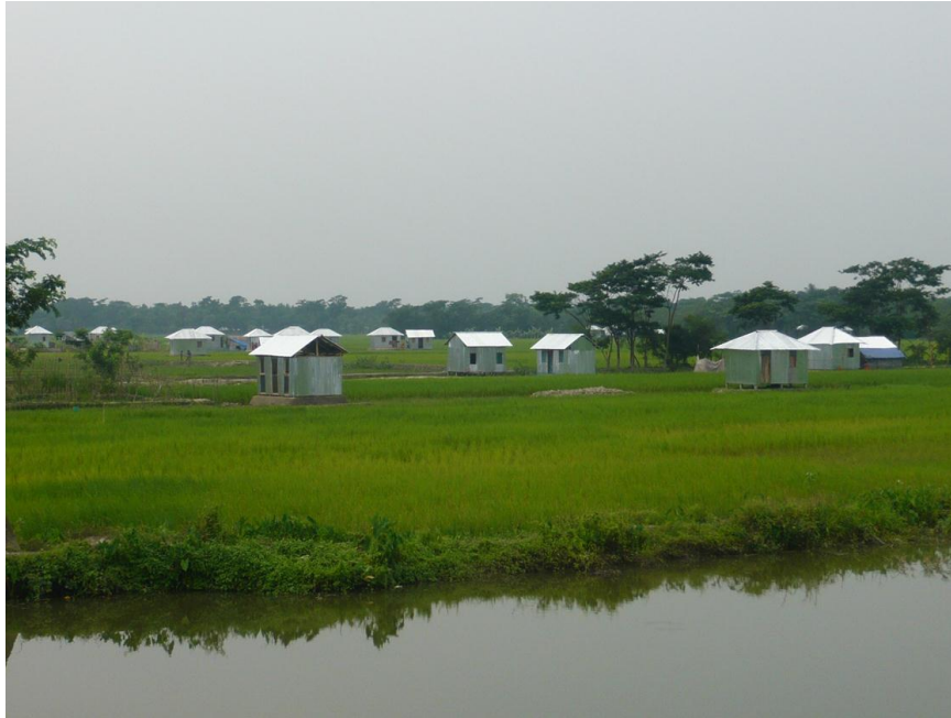
Figure 1. Constructed houses by NGOs in paddy field after the cyclone Sidr 2007
