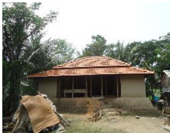
Figure 10. Photograph of completed house in Assasuni, Satkhira
