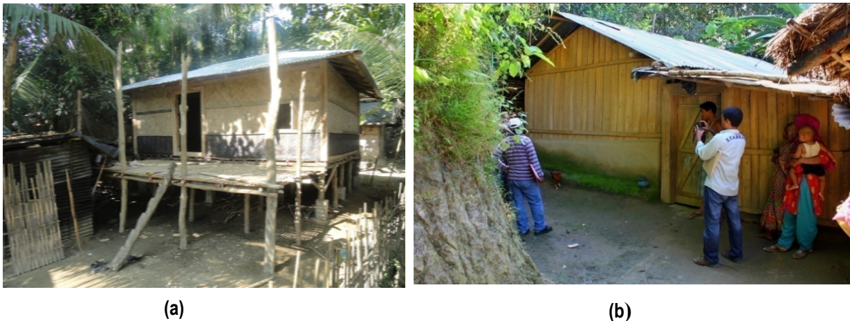
Figure 11. (a) Photograph of machan house and (b) house on ground in Bandarban
