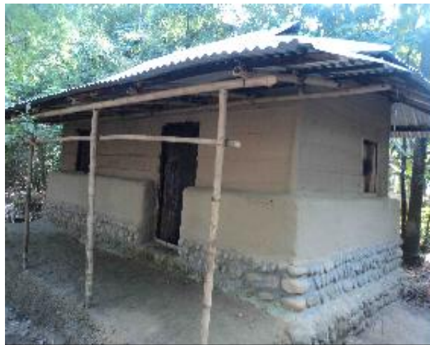
Figure 7. Photograph of completed half walled house with stone plinth in Kanaighat, Sylhet
