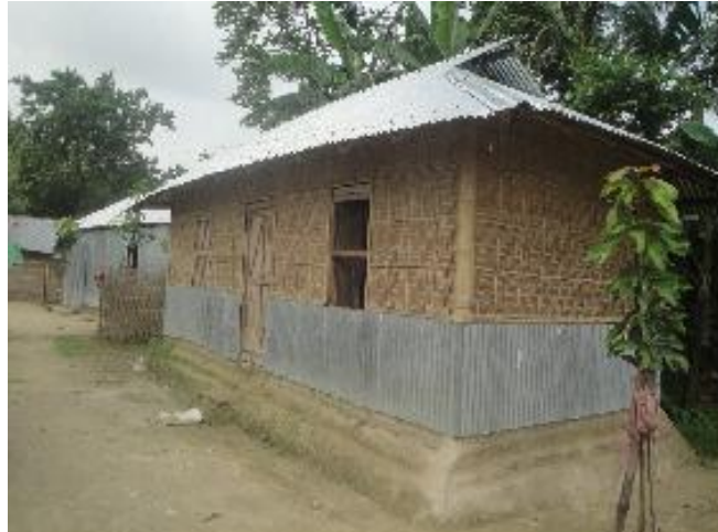
Figure 6. Photograph of completed house in Gaibandha
