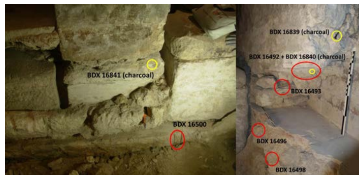
Fig. 1 The south-eastern angle of the central chapel with marked samples from the first intervention in the crypt: BDX 16496, BDX 16498 and BDX 16500 correspond to the Late Antiquity mausoleum, BDX 16493 and BDX 16492 to two consequent construction phases
