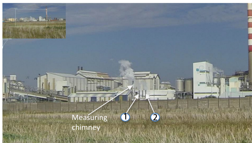
Figure 7. Location of other measured sources of ammonia (chimneys 1 and 2) near the measured plume (view from the GoPro camera in position 2).
