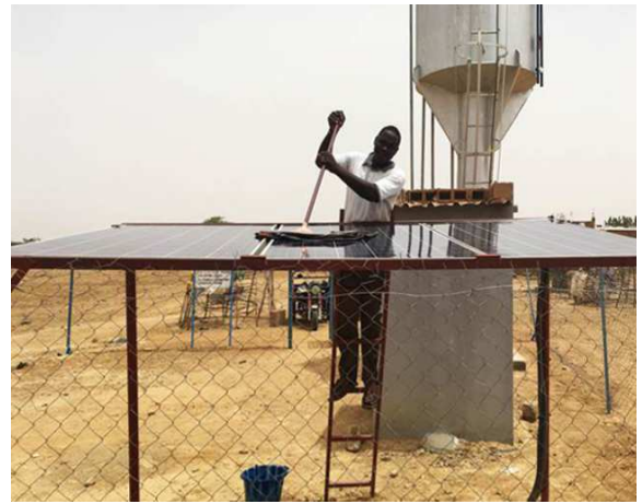
Figure 2. Cleaning intervention on the photovoltaic array
