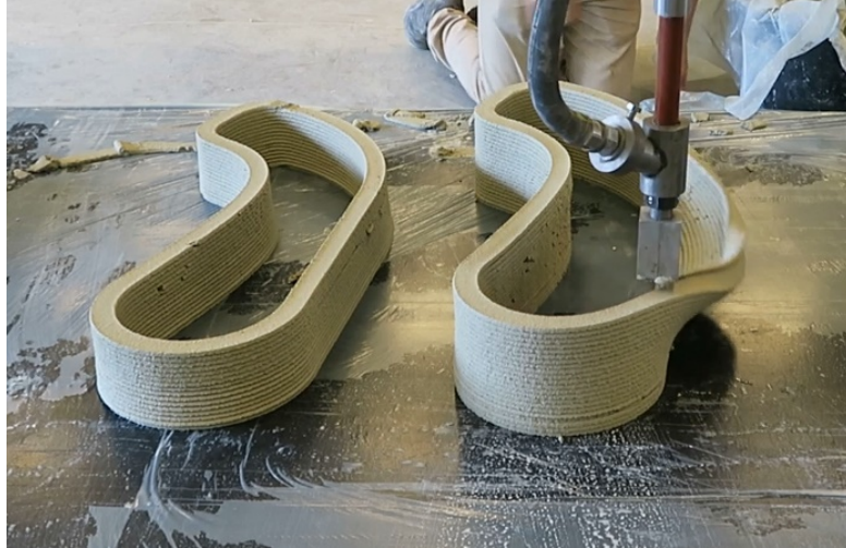
Figure 9. Elastic buckling during a 3D printing process.
