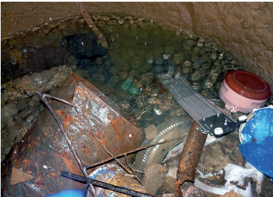
Fig. 14. The bottom of PU211 at a depth of 31 m, shows the impossibility of collecting ceramics
