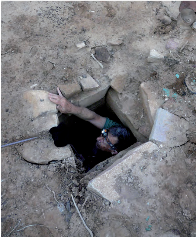
Fig. 13. Man hole 566, of a diameter of 0.6 m, is not easy to explore. It has allowed us to determine the altitude of the qanât
