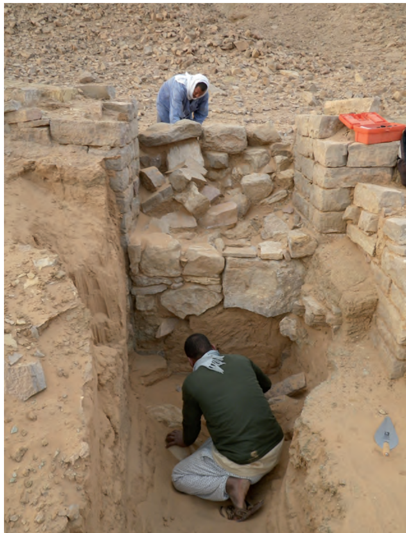
Fig. 20. Excavation of the gate in progress, looking south (DJ2013a0197B)
