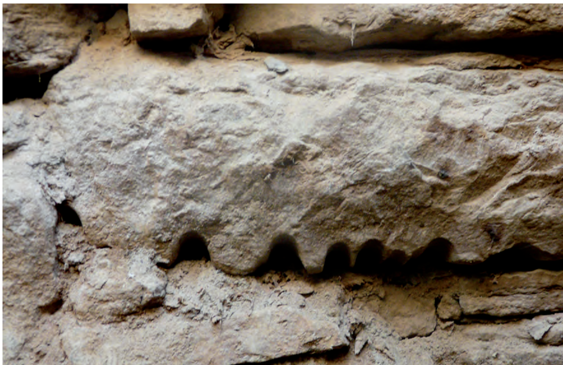
Fig. 17. Reuse of striated stone of a curbstone in the reconstruction of a well.
