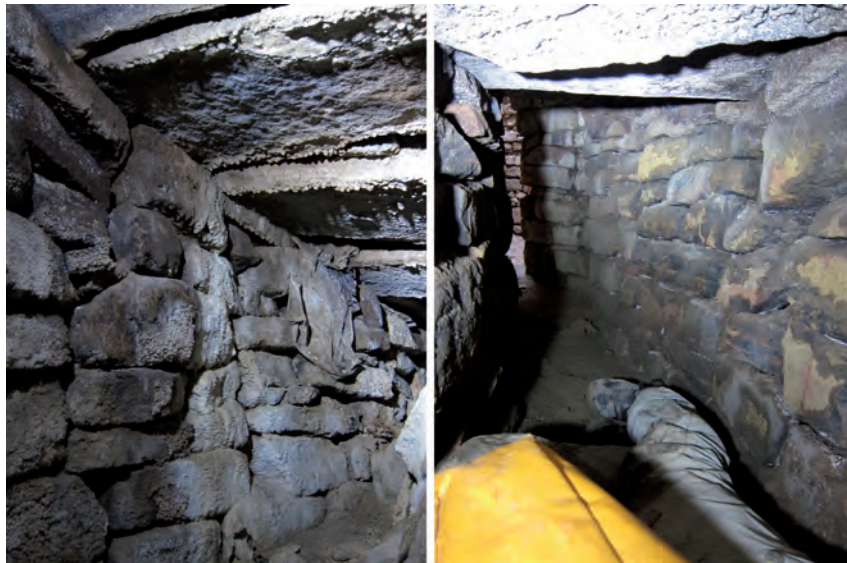
Fig. 15. Qanât masonry, of low rise and a challenging course
