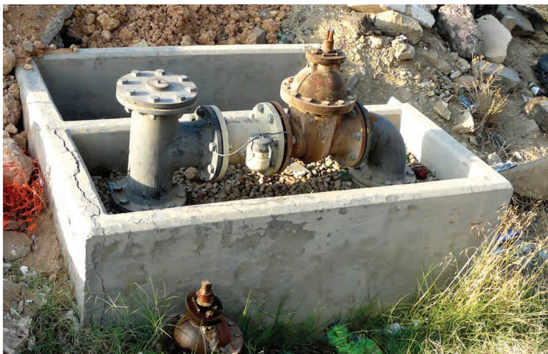
Fig. 12. New system fed by big pumping stations
