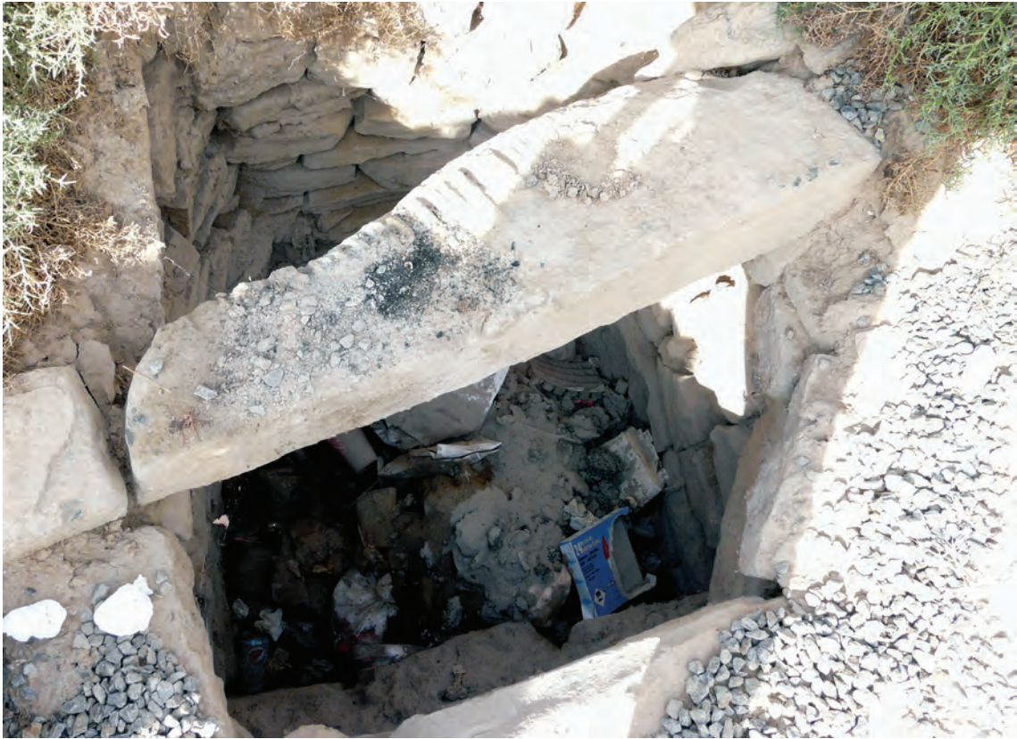
Fig. 31. Sight hole 150, located near ‘Ayn al-Âmir. It would be interesting to empty it of collapse and infilling to know the qanât’s elevation
