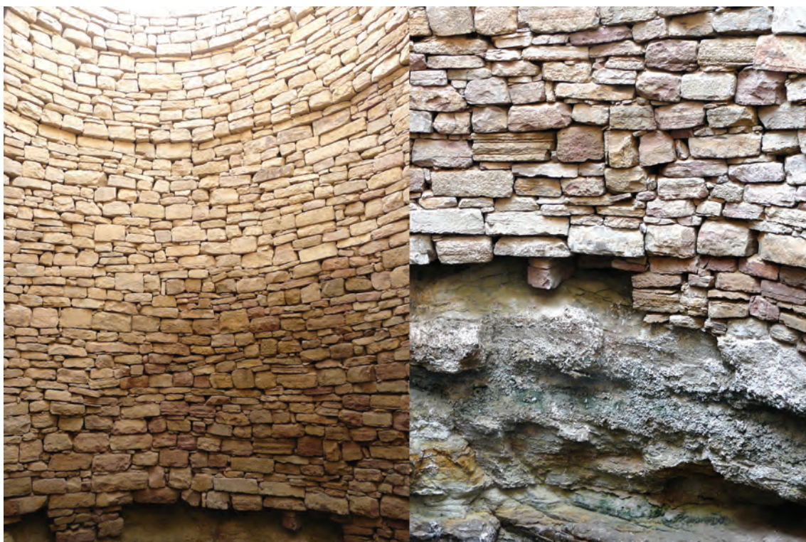
Fig. 20. This photograph taken in well PU178, shows the extent of the built part of wells and the technique of use of stones with no bonding, without any mortared joints. Curiously, the course of the built section leaning on the Sha'iba rock, seems made of small stones. Siltite stones in pink tones, forming beautiful limestone slabs, can be distinguished
