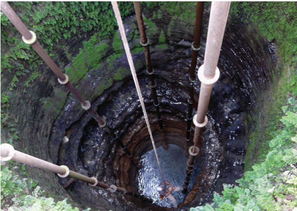
Fig. 11. At well PU211, there are six pumps, no doubt for irrigating the fields of six different landowners. One of the pipes has disappeared
