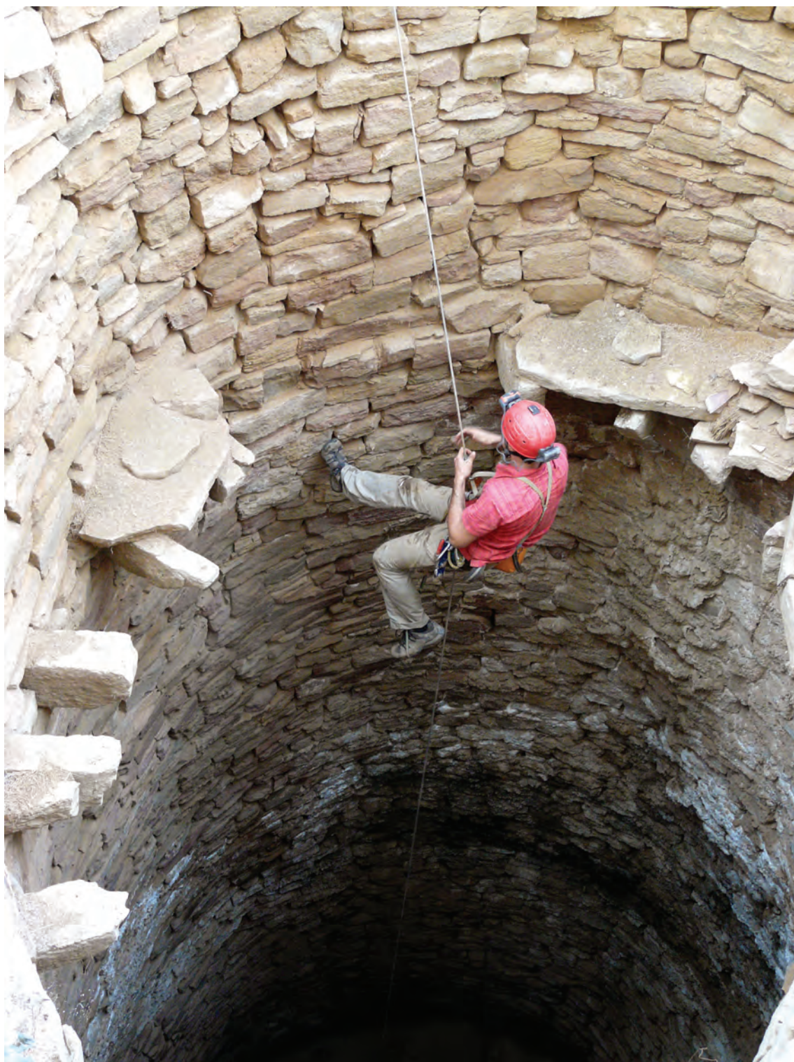
Fig. 33. Well PU184 is the only one where we found corbels which supported a balcony
