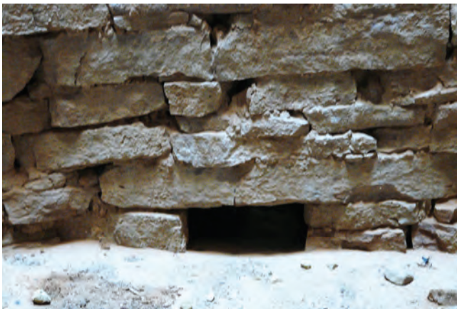
Fig. 32. One of the sight holes opening at the base of Bîr Hasya and which would be interesting to empty of sand
