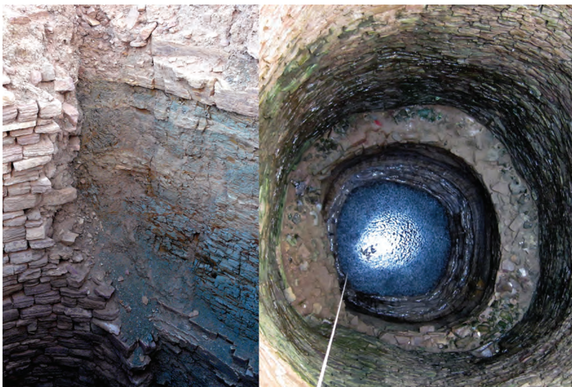
Fig. 15. The friable rock in the photograph to the left shows why the top of the well was constructed. To the right, one can see the change in rock, with the constructed part in the Qasr member and that dug in the Sha'iba member
