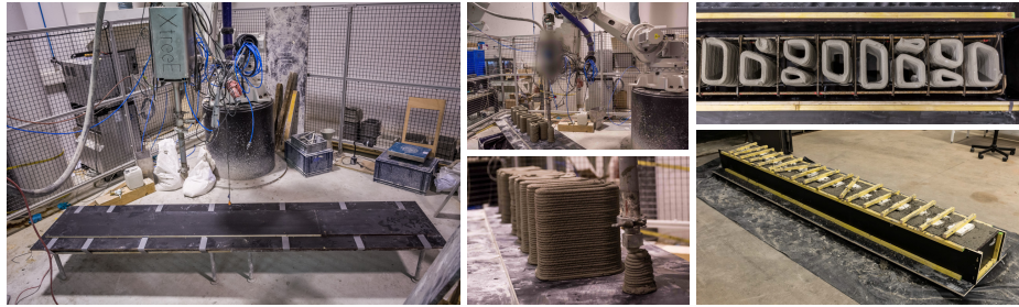
(a) Fabrication of the prototype with, from left to right, preparation of the printing cell, printing of the formwork, final preparation of the formwork and, pouring of the concrete
