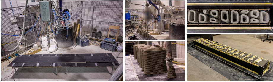
(a) Fabrication of the prototype with, from left to right, preparation of the printing cell, printing of the formwork, final preparation of the formwork and, pouring of the concrete
