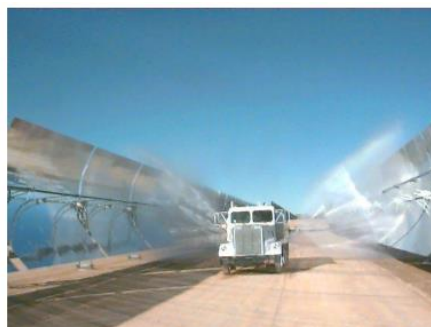
Figure 3: The traditional deluge method in operation
