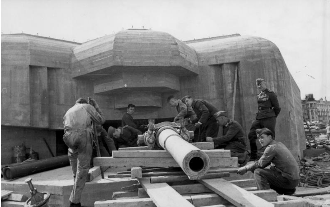
Fig. 1: Constructing an Atlantic Wall bunker, Northern France 1943 by Müller (Photo copyright: CC-BY-SA 3.0 Bundesarchiv, Bild 101I-294-1531-14 / Müller) https://commons.wikimedia.org/w/index.php?curid=5476912
