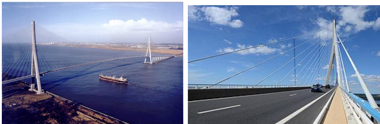
15 16 (a) (b) 17 FIGURE 1 Bridge of Normandy, (a) aerial view from the south, (b) view of the deck.
