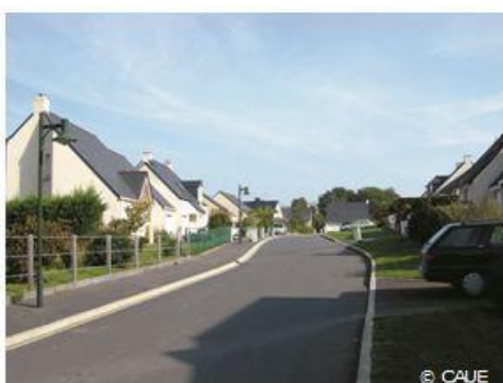
Fig. A13. Housing estate
