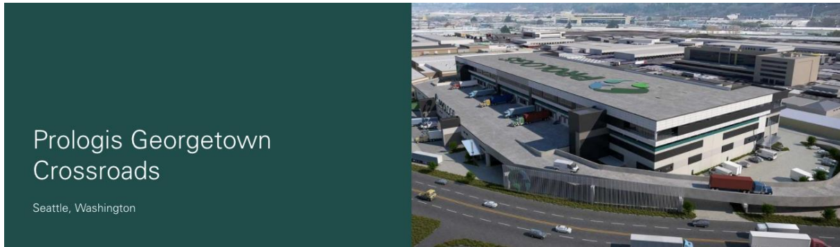
Figure I.9: First Prologis multi story warehouse in the US Source: Prologis
