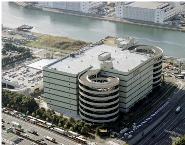
Figure I.8: Seoul Integrated Freight Terminal, Seoul, Korea (built in 2015) Photo: L. Dablanc, 2016
