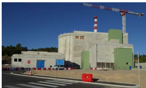
General view of Reactor Building and Auxiliary unit building (Fall-2016)
