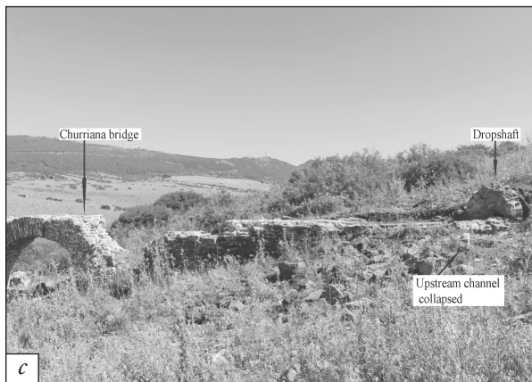
Fig. 2 - The Dropshafts of the Aqueducts of Baelo Claudia and the comparison with the Valdepuentes Aqueduct of Cordoba. a: Dropshaft at the Realillo aqueduct excavated in 2016; b: Dropshaft ahead the Chorrera bridge (aqueduct of Punta Paloma); c: Dropshaft ahead the Churriana bridge (aqueduct of Punta Paloma); d: Dropshaft ahead the Valdepuentes bridge (aqueduct of Cordoba). [copyright: Laetitia Borau]
