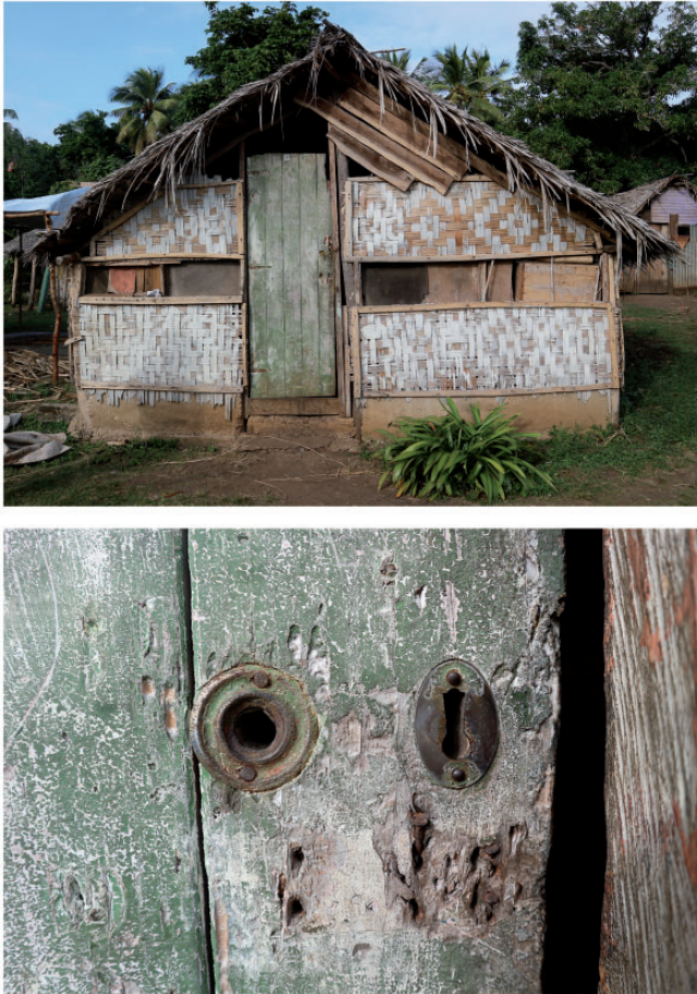
Figure 3. Door from the historical mission church integrated into a 'traditional' Aniwan house (above); detail of the original lock (below).
