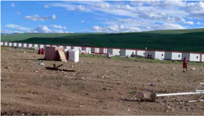
Figure 14.5 The complex of prefabricated metal quarters
